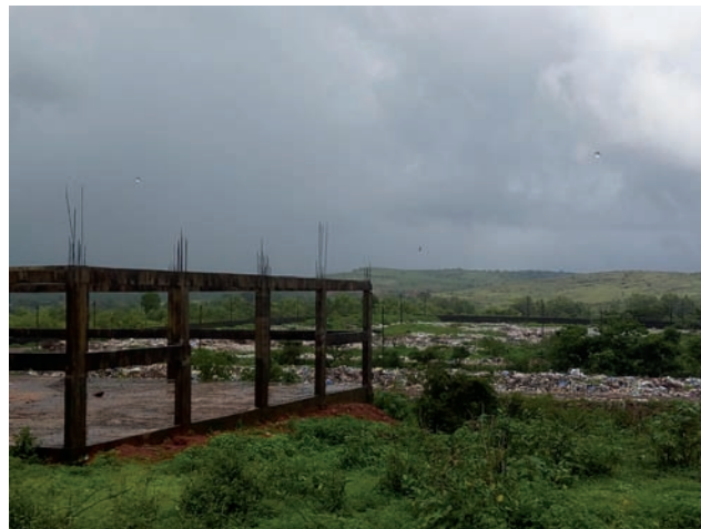
Waste processing unit under construction at the Bhatkal landfill site
