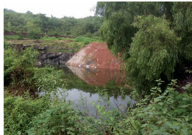
Monsoon rainwater and landfill leachate accumulated at the Ankola landfill site
