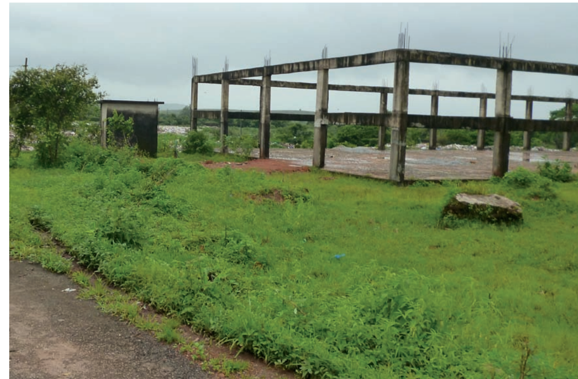
Bhatkal waste processing unit under construction
