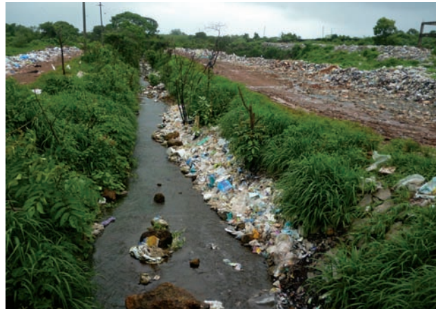
Landfill with no proper compaction and grading to prevent infiltration during monsoon in Bhatkal
