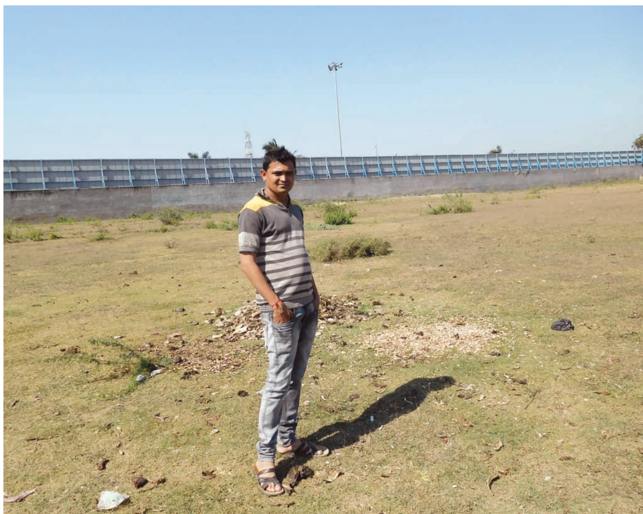
A community member standing near the extended boundary walls—now 9 metres high—around the facility's coal storage area Photograph: Vijay Rathod
