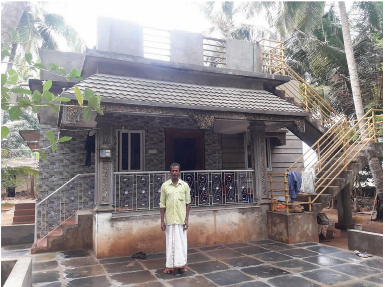
Somnath Naik standing in front of his newly constructed house—he earlier had a mud house Photograph: Maruti Gouda
