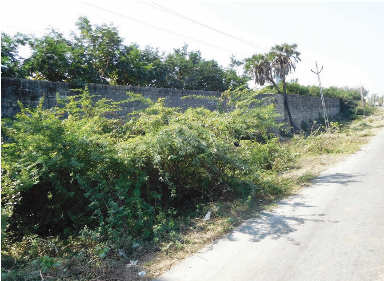
Improved green cover around the boundary walls of the facility, in compliance with the Coal Handling Guidelines Photograph: Vijay Rathod
