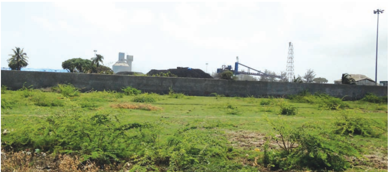
Coal stacks visible well above the boundary wall that is shorter than 9 metres, the height prescribed by the Coal Handling Guidelines Photograph: Vijay Rathod
