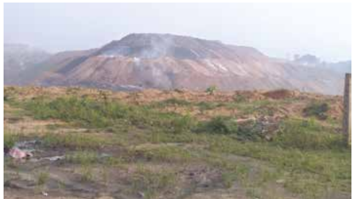
Coal fire in the OB Dump of Kulda OCP
