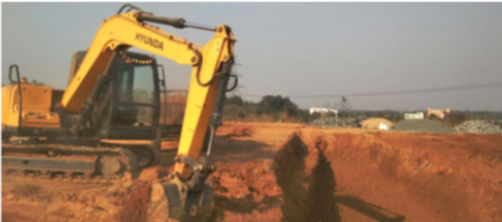
Figure 3: Land excavation work in progress at Dhenkanal
