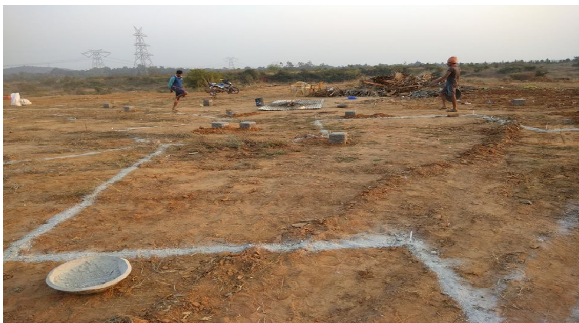
Figure 4: Initial stages of commencement of construction of the FSTP at Dhenkanal
