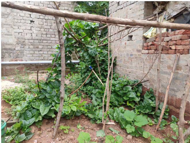
Figure 21: Extra Pipes laid for HH Tap connection
