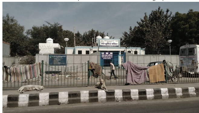
Photo 11: Newly built toilet complex on Maharishi Valmiki Marg between Hanuman Camp and D Block JJC in Mangolpuri
