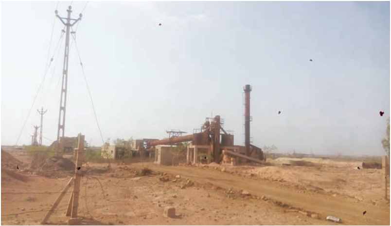
The Somnath Bauxite Plant
