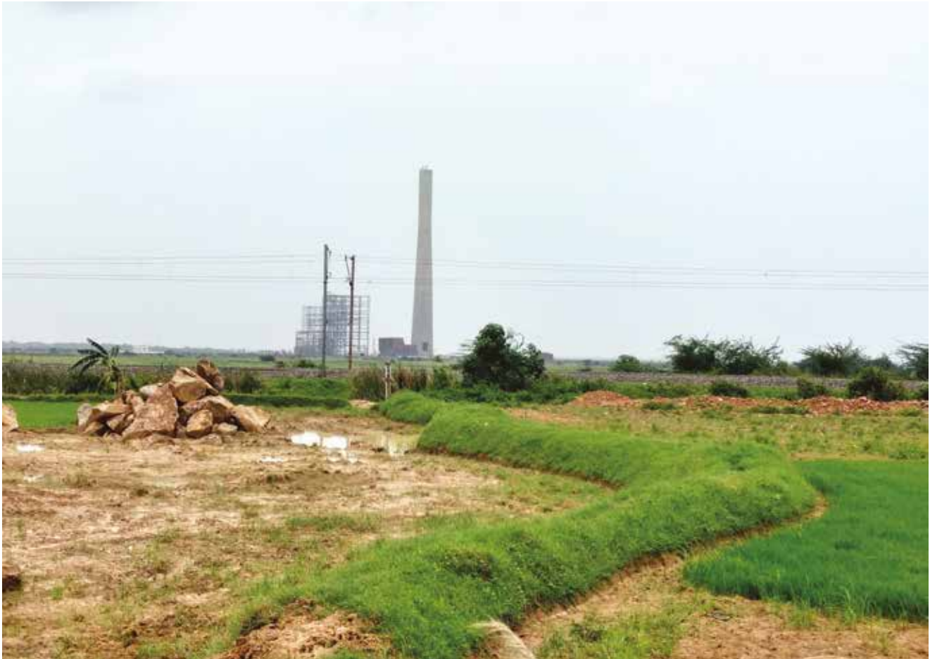
Bhavanapadu power plant, Andhra Pradesh
