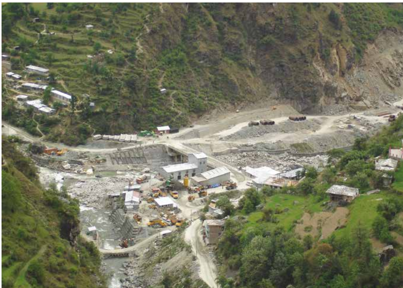
Hydropower project under construction in Himachal Pradesh
