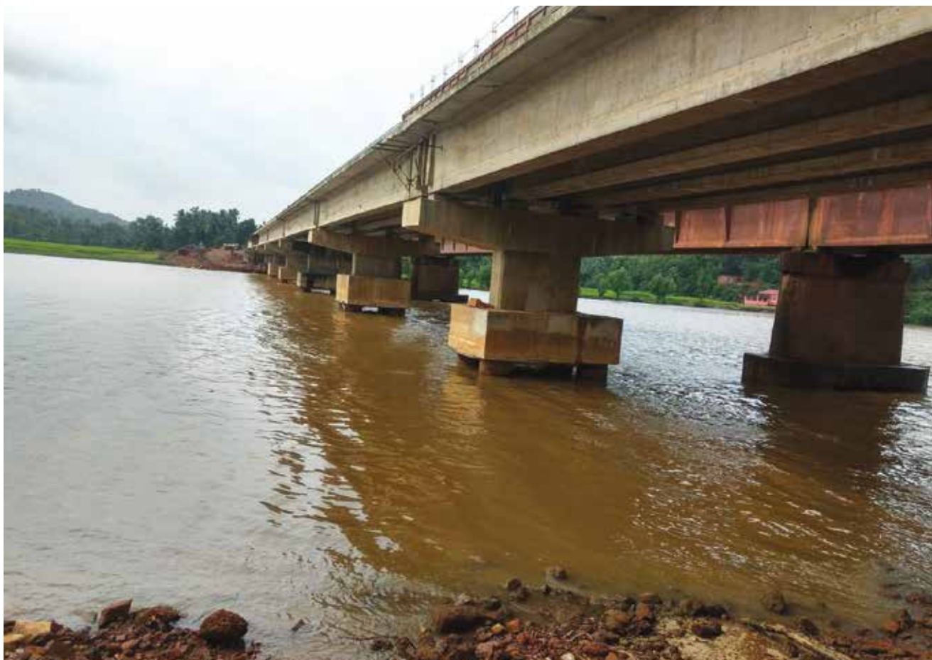
Bridge built on Gangavalli River as a part of NH 66 road expansion. Sand dumping for construction of this bridge caused the salt water intrusion at Chandumata
