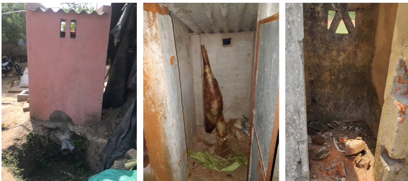
Figure 3 Clockwise list of figures (from top left): Individual toilet missing an on-site sanitation system in Puri; dysfunctional toilet at an AWC in Angul; unused individual toilet facility being used for storage in Debagarh
