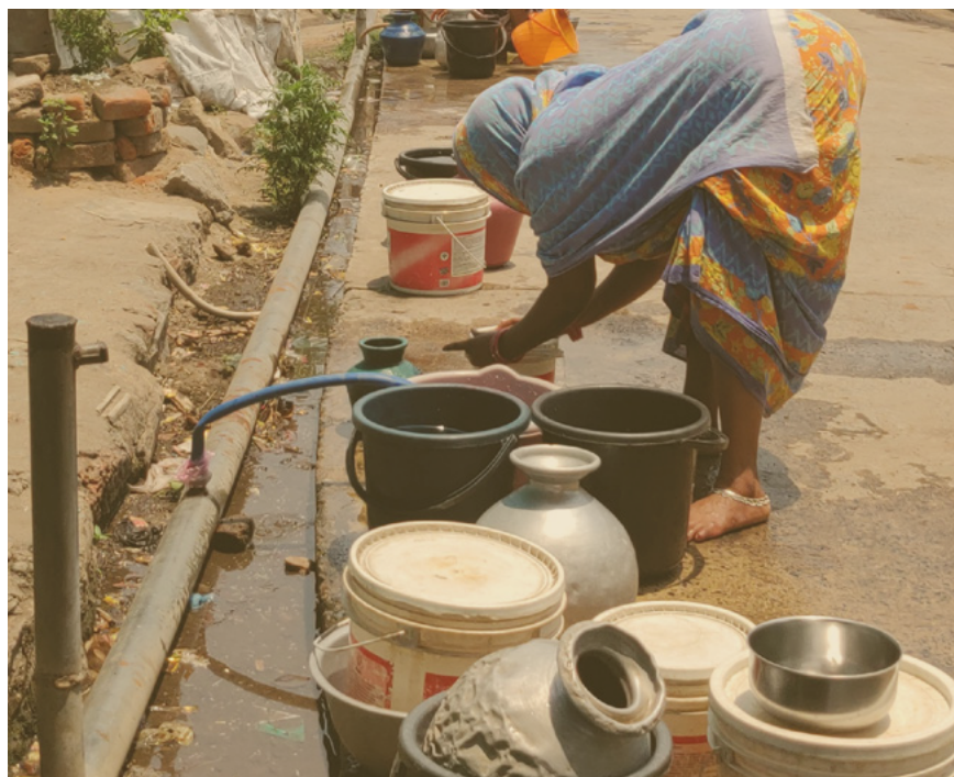
Standpipe in Angul Angul district
