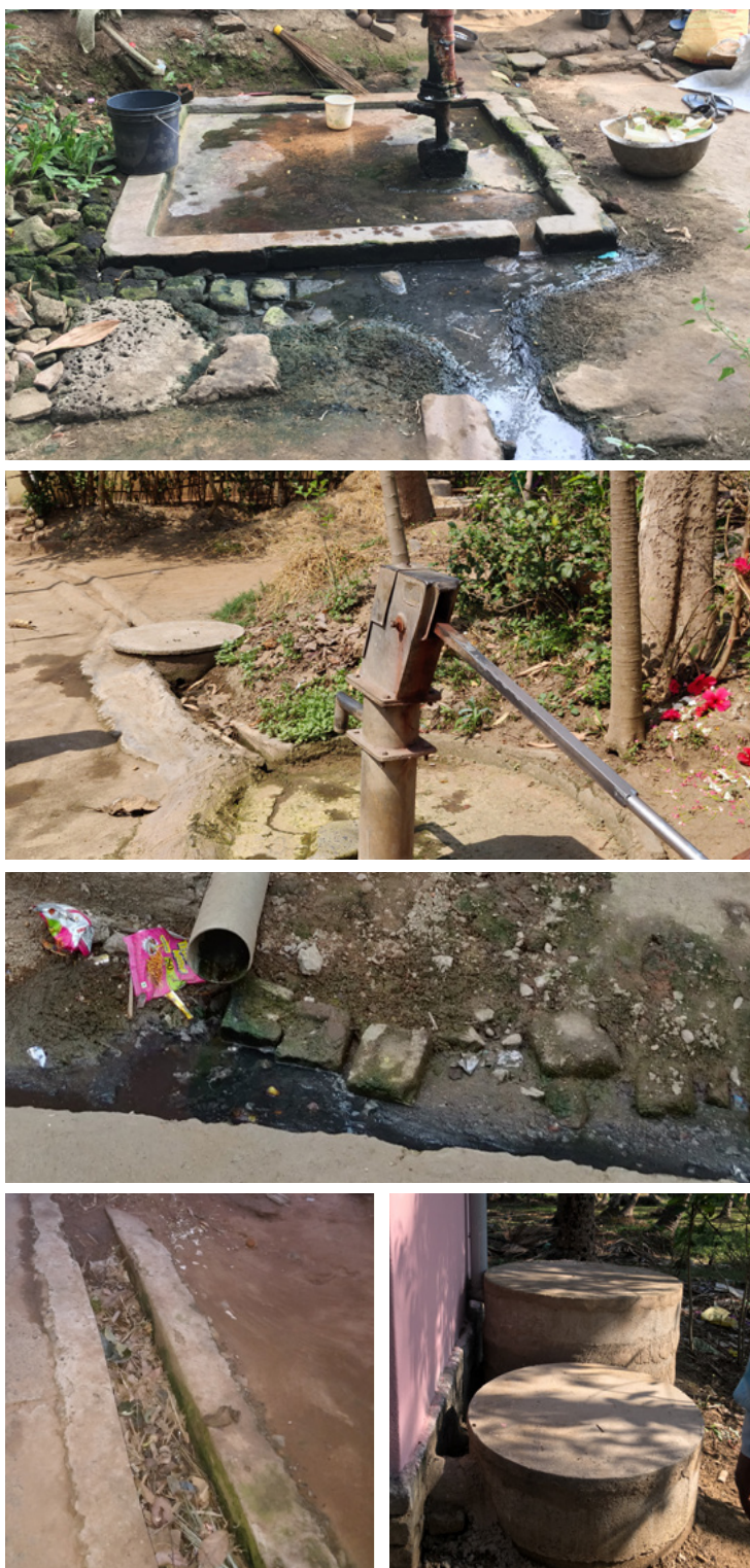
Figure 5 Clockwise list of figures (from top left): Stagnation of sullage within household premises in Puri; Public handpump connected to a soak pit chamber in Angul; sullage discharge to a stormwater drain in Angul; a system of two individual single pits for blackwater and sullage management respectively in Puri; choked drain in Debagarh
