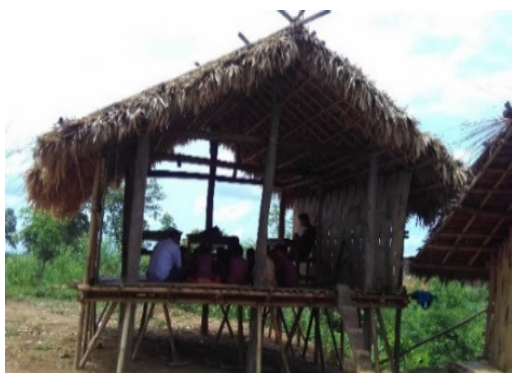
Picture 2: School run in bamboo shed
