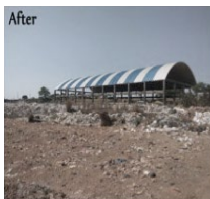
Landfill site cleaned up and managed by Municipal Authorities as per Solid Waste Management guidelines due to efforts of Program's field team in Karnataka
