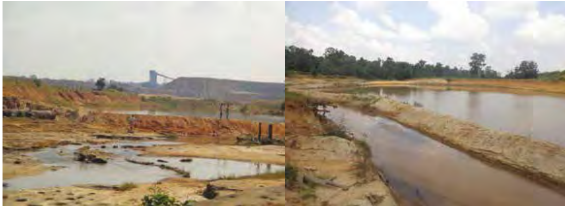
Reservoir for waste water from the coal pit- created by diverting the flow of the nala at Ghatbarra
