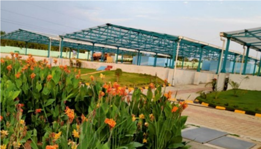
Sludge drying bed-based FSTP
