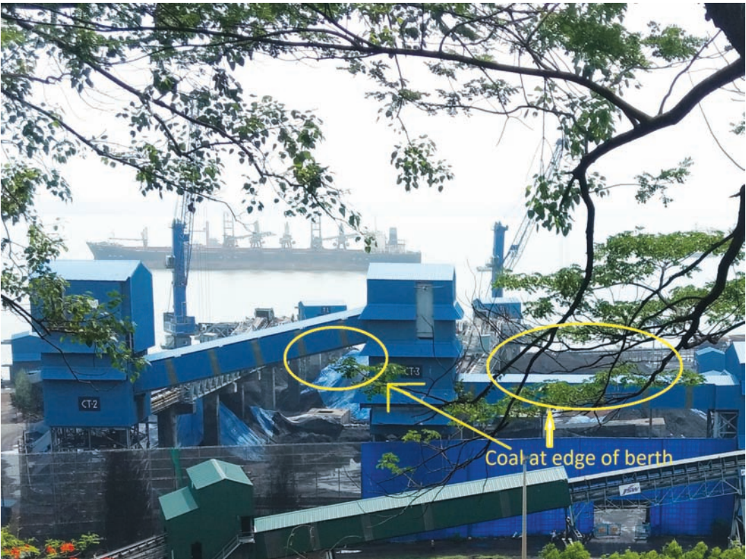
Unloading on Berth 7 May 2018; Pic credit: Tania Devaiah
