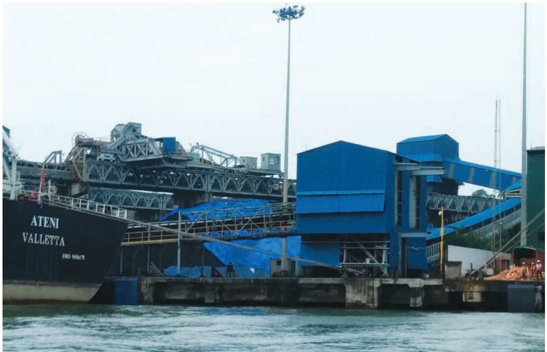
Unloading on Berth 7 water's edge July 2018; Pic credit: Tania Devaiah
