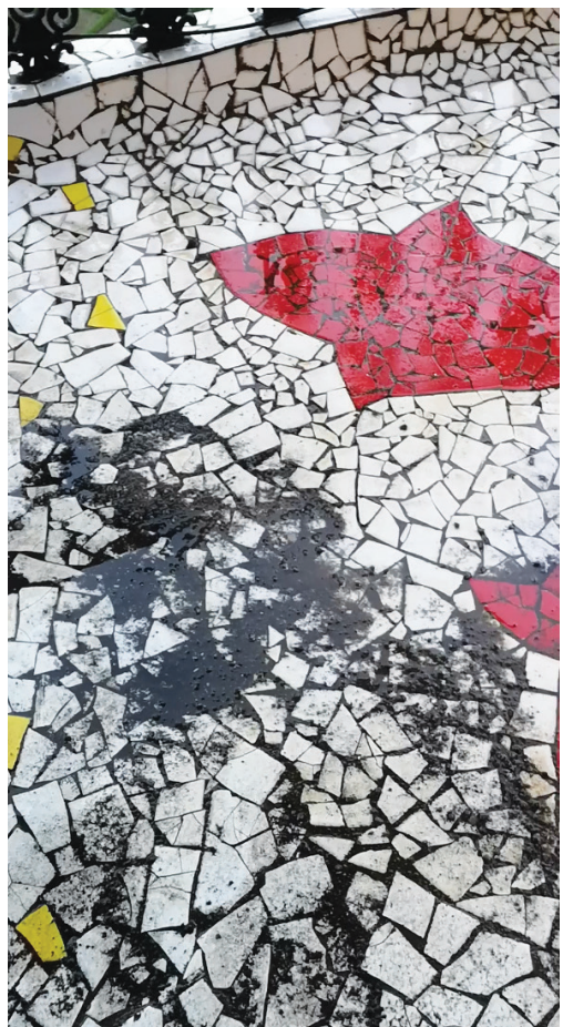
Coal dust on the balcony in the residence of Mrs. Ema Mascharenhas, July 2018 Pic credit: Goa against coal
