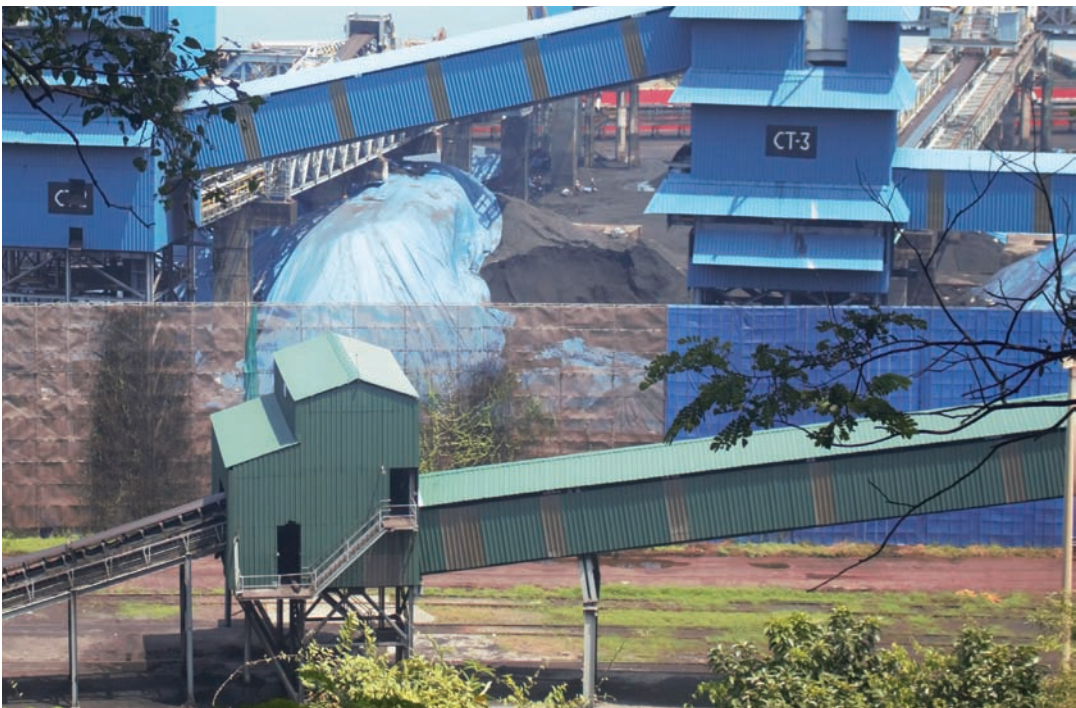
Lack of creepers on windscreen and only partially covered by fabric/tarp, Oct 2018; Pic credit: Tania Devaiah
