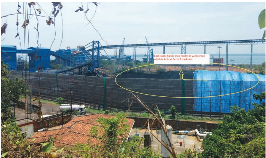
Coal stack higher than the height of windscreen, July 2018; Pic credit: Tania Devaiah
