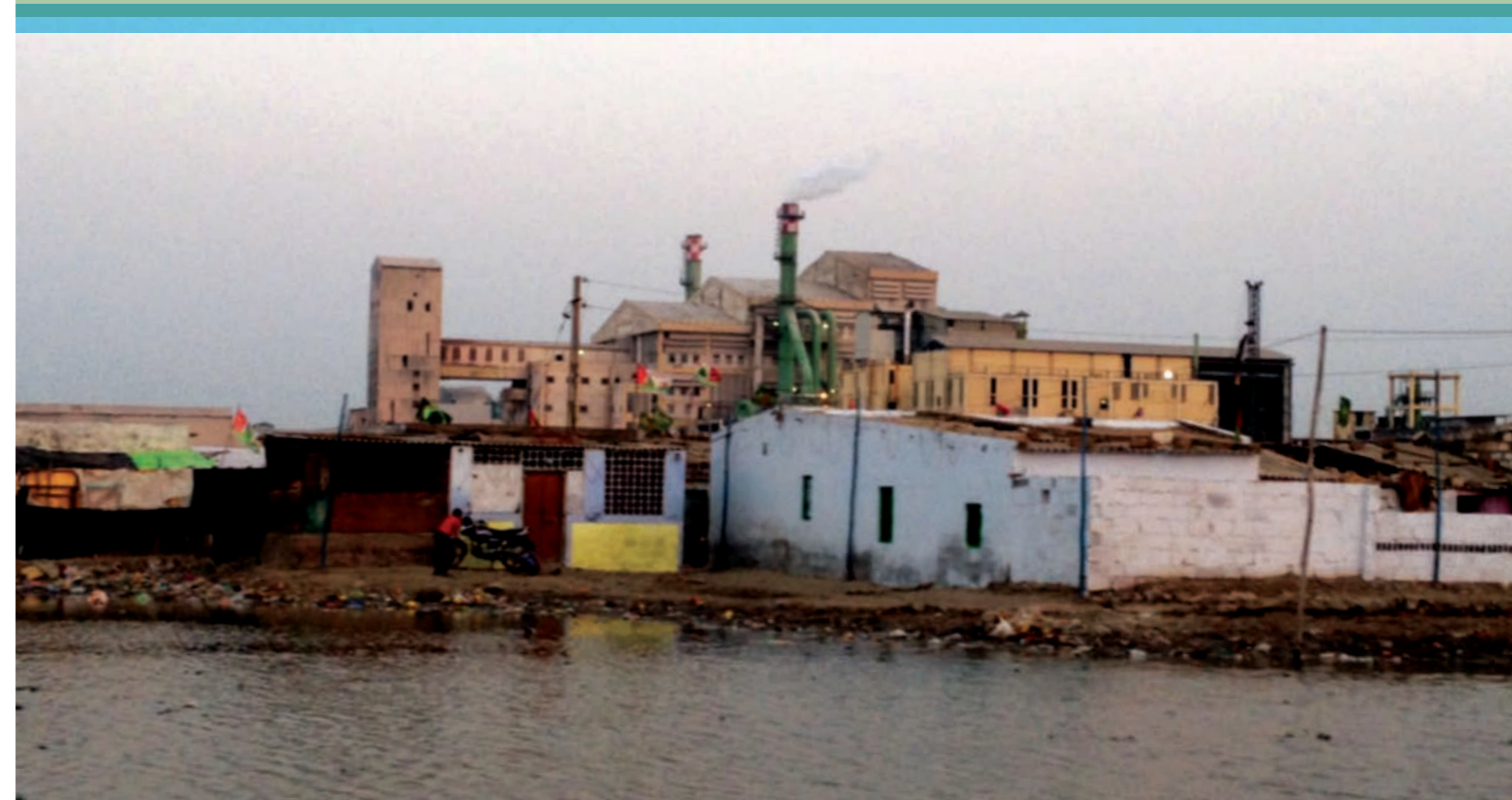
The chemical storage plant in the No Development Zone in violation of the CRZ law, Gujarat
