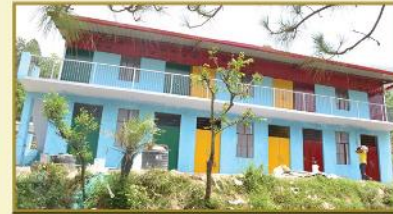
The Brightland School, which was rebuilt as a WASH-friendly school with the help of GIWA after it was destroyed by floods
