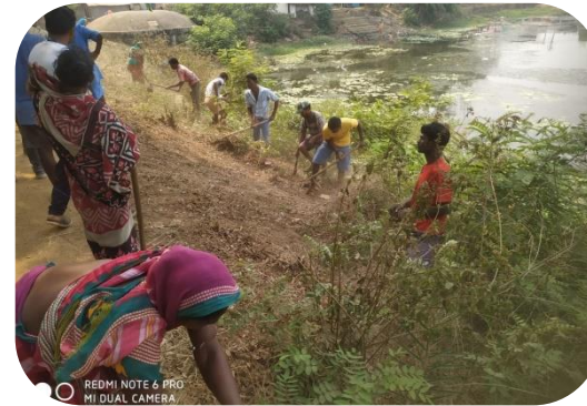
WATER BODY RENOVATION
