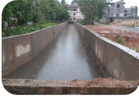
DRAINAGE AND SEWERAGE WORK
