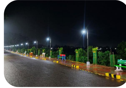
PAVERED WALKING TRACK
