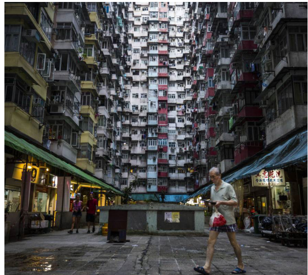
Figure 9: Affordable housing in Hong Kong
