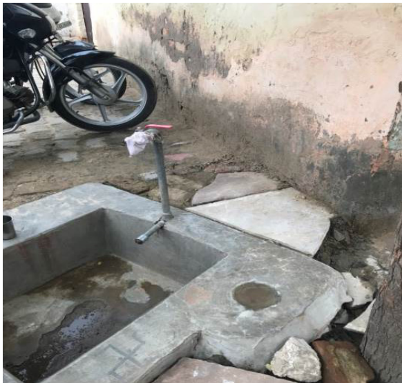
Picture 14: Household water stand post; concrete structure is constructed to stop water spilling over to the street, Jaipur
