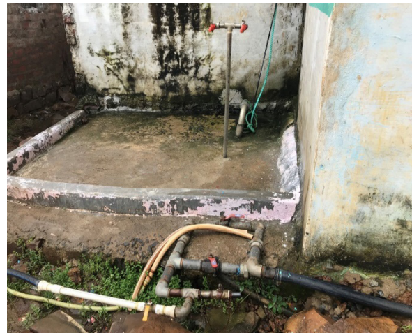
Picture 4: Water pumping point; pipelines extended to individual households in Anandpura, Bhopal
