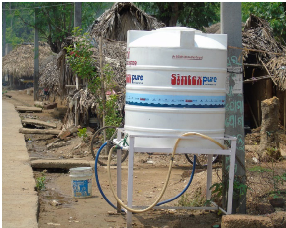
Picture 16: Due to the efforts of SSCs, water tanks like this are installed in Radha Raman Pada in Angul that do not have piped water supply
