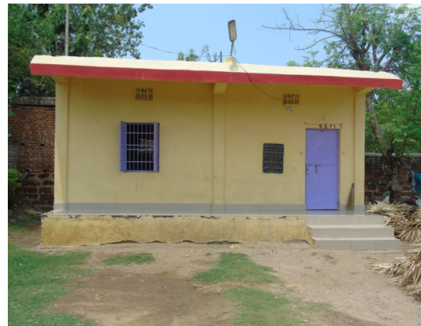
Picture 17: Due to the efforts of Slum Sanitation Committee, a community hall was constructed in Radha Raman Pada in Angul
