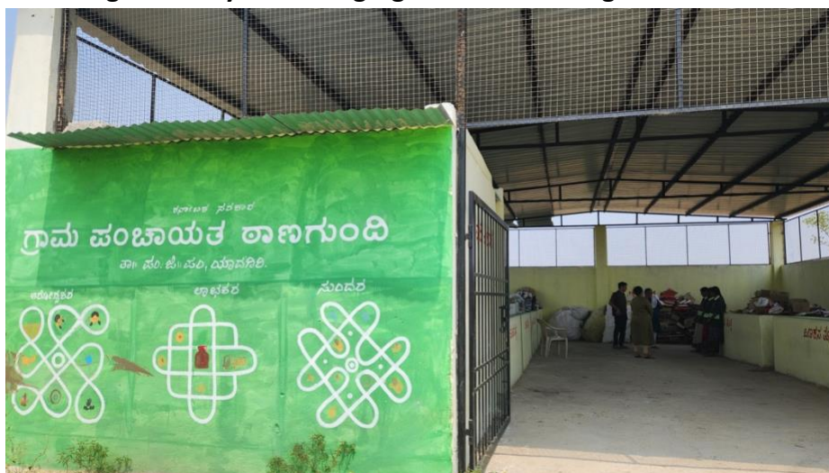
Figure 8: Dry Waste Segregation Unit in Yadgir GP
